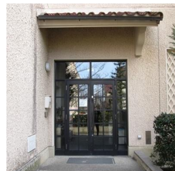
door to Building IV, guard window
